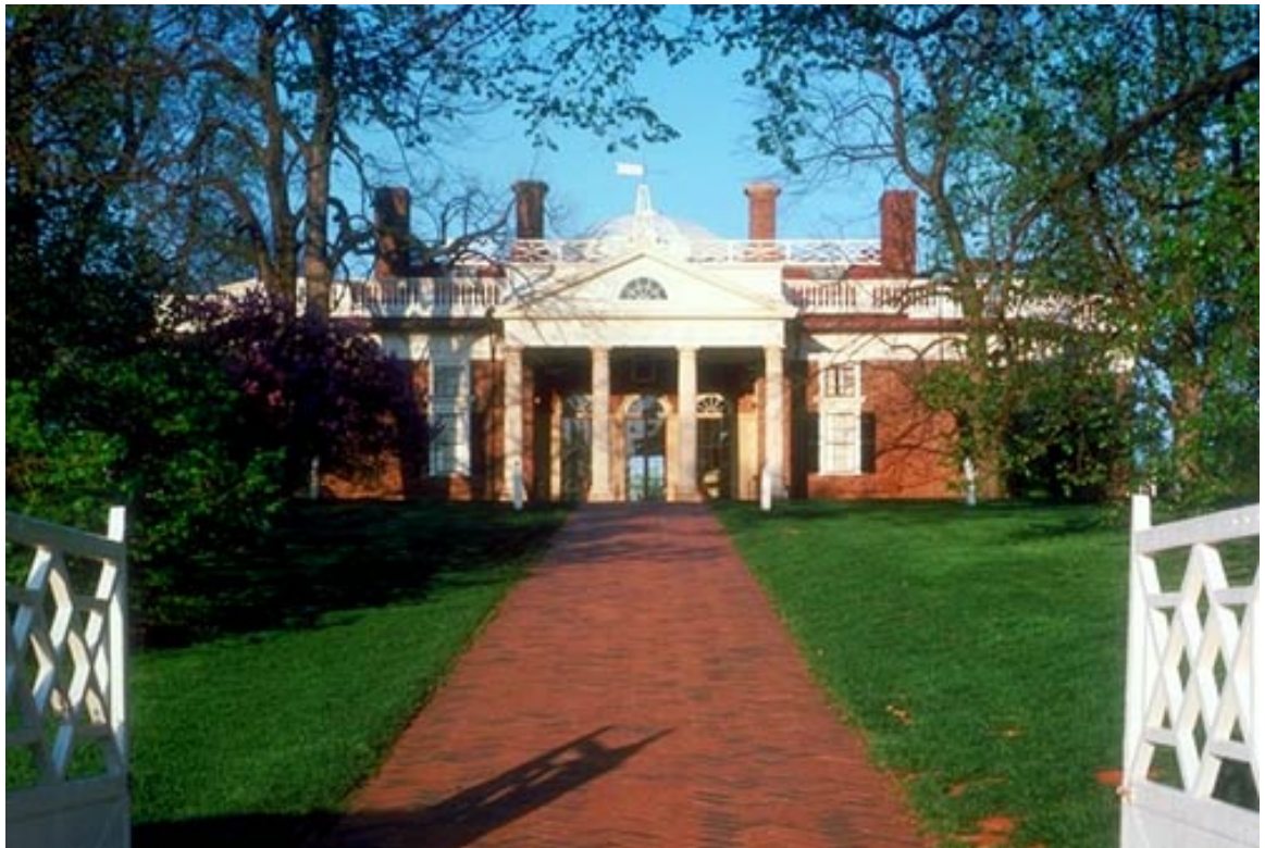
Jefferson's Monticello, east front
